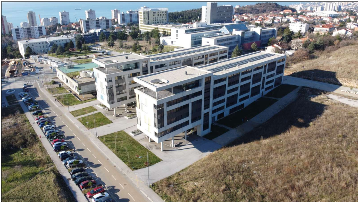
Student dormitory Trsat: pavilion 1 and 2
