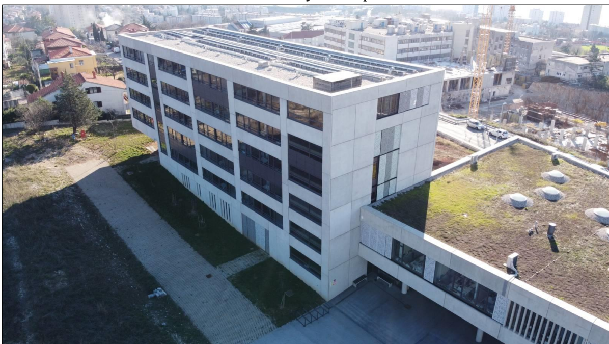
Student dormitory Trsat: pavilion 4
